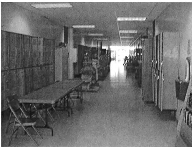
Semon Hall Interior Corridor
